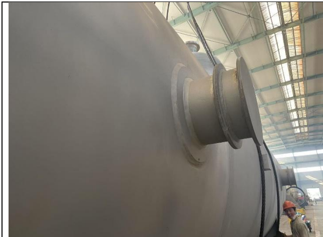
Blasting inspection (TAG-01)
