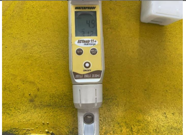
Blasting inspection (TAG-01)
